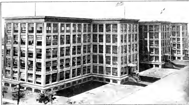
FIG. 5. REAR VIEW OF FIG. 3. SERVICE INSTALLATIONS AND STAIRWAYS ARE IN THE WINGS TO KEEP THE MAIN BUILDING CLEAR AND AVOID CONGESTION OF TRAFFIC.
